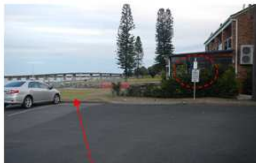
Image 3 – Install missing “90 degree parking – Front or Rear to Kerb, Vehicles under 6m only” (to left) and No Parking (to right) signs. Remove two unnecessary signs (circled)
