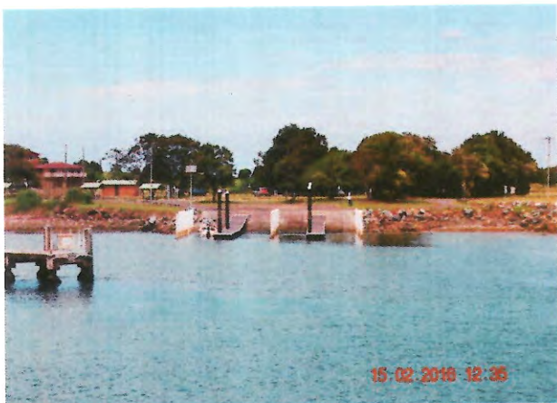
4 Lane boat ramp with condemned jetty (left)
