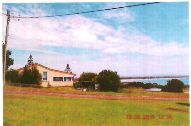
Crowdy School deteriorating (room to move)
