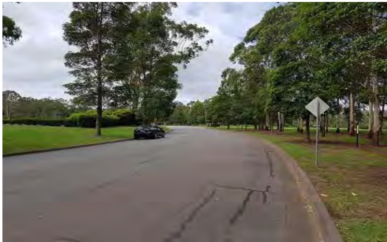
Photo Plate 3 – The Boulevard looking south toward Blackhead Road
