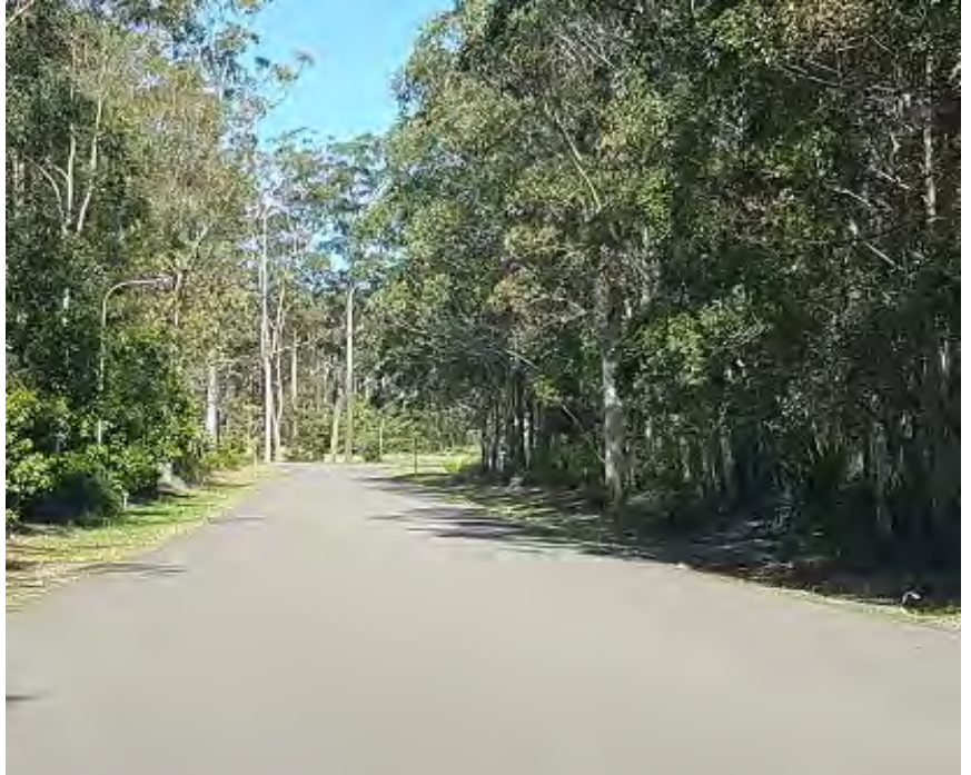
Photo Plate 4 – Grangewood Avenue looking east toward The Boulevard
