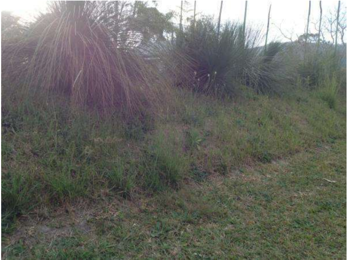
Photo 3: An earth mound is already constructed near the boundary and acts as an acoustic barrier.
