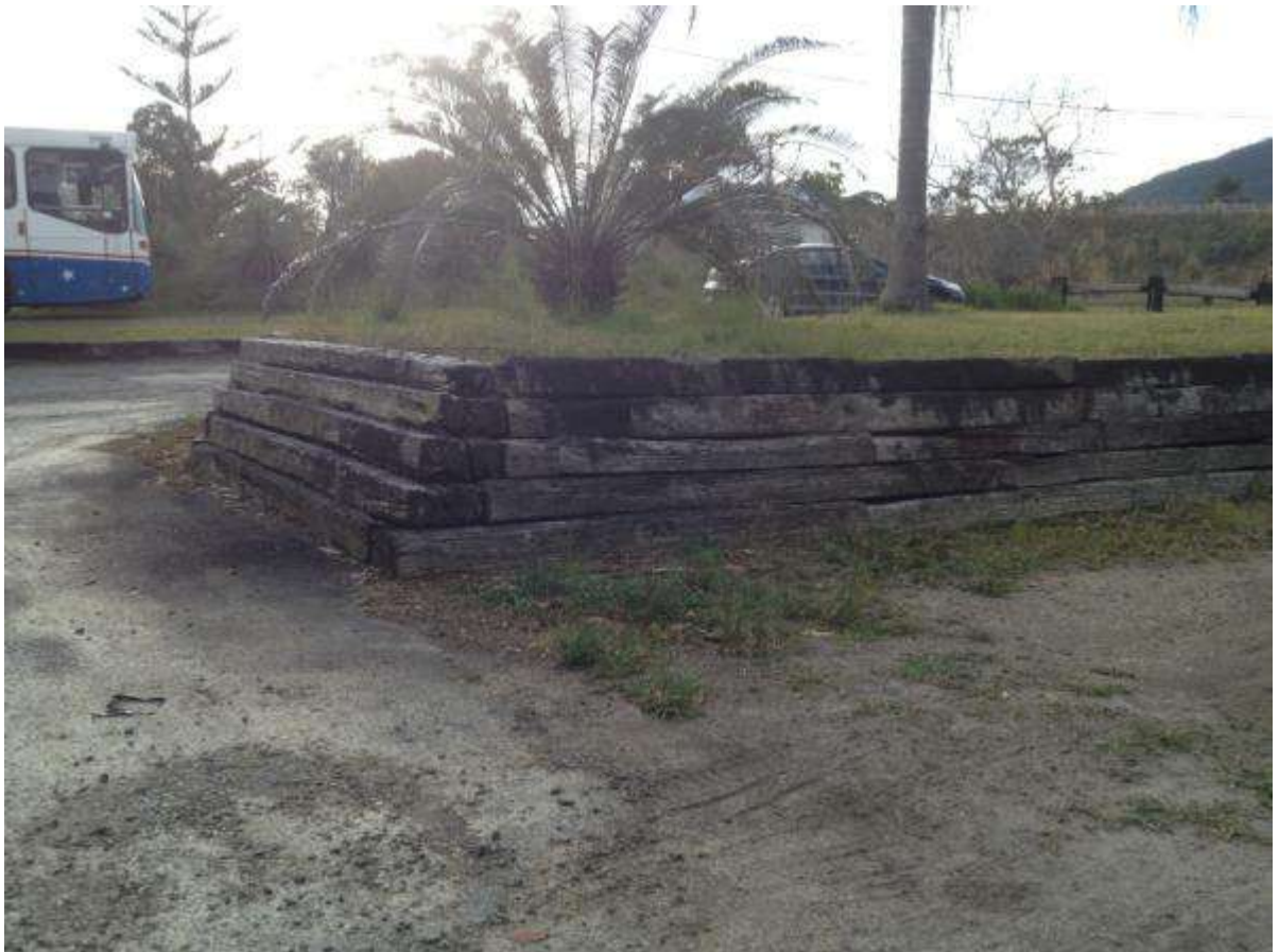
Photo 4: Existing low retaining walls will help block noise.
