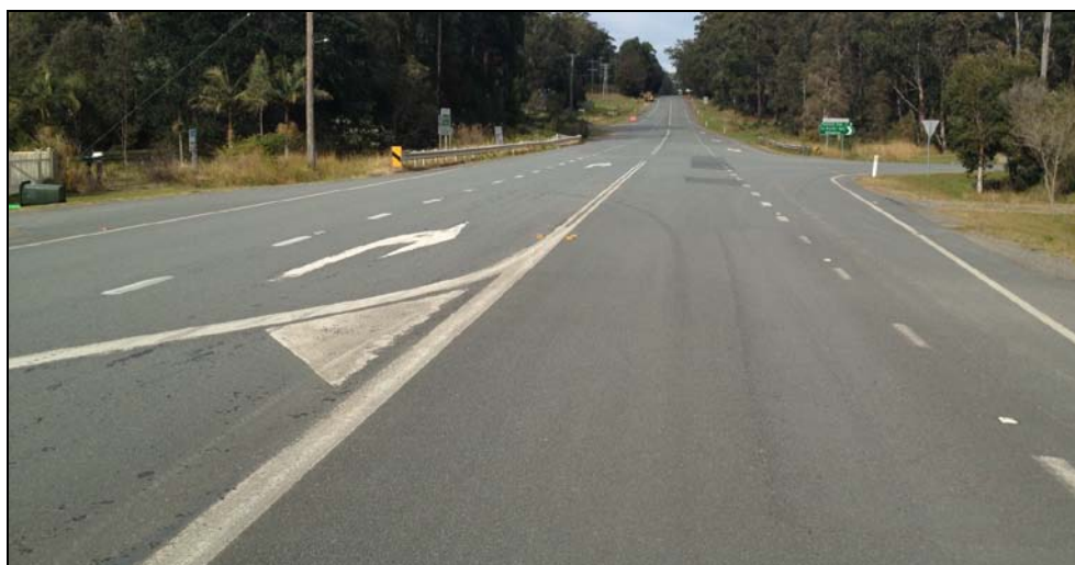
FIGURE 2.4: JOHNS RIVER RD/KOOLYANGARRA RD INTERSECTION LOOKING SOUTH
