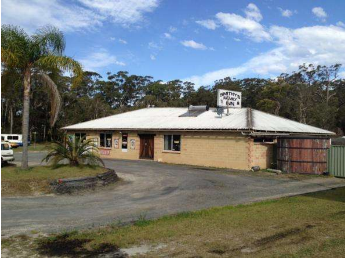
Photo 1: The proposed Fuel Outlet will be attached to this side of the Tavern.
