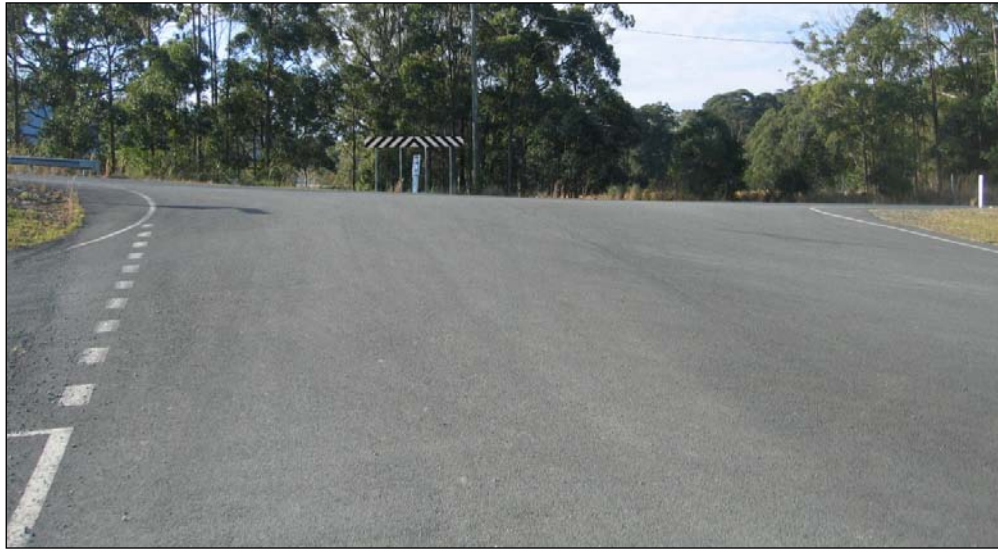
FIGURE 2.2: SITE ACCESS ROAD LOOKING NORTH TOWARDS JOHNS RIVER ROAD
