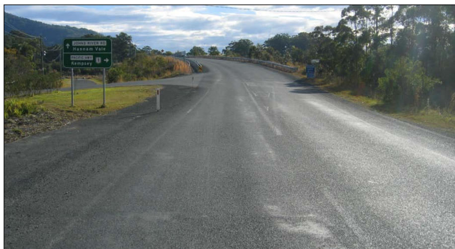
FIGURE 2.1: JOHNS RIVER ROAD LOOKING WEST SHOWING SITE ACCESS INTERSECTION
