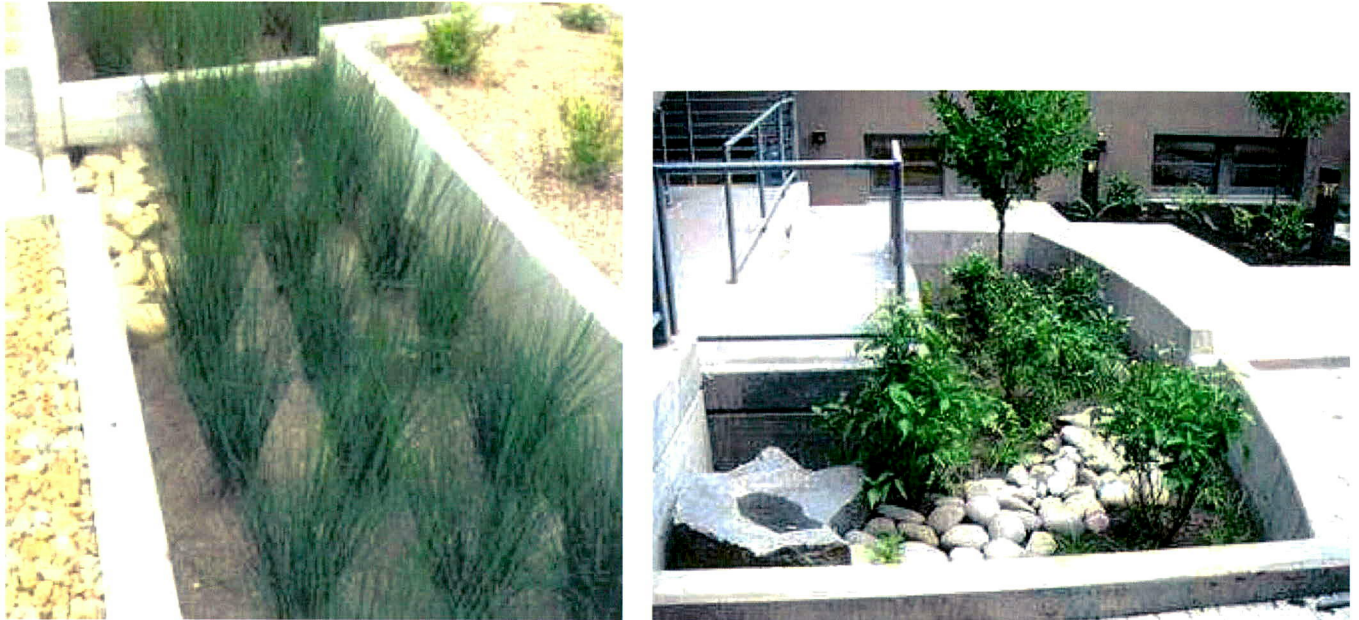
Figure 3: Indicative Planter Box style Bioretention Basins
