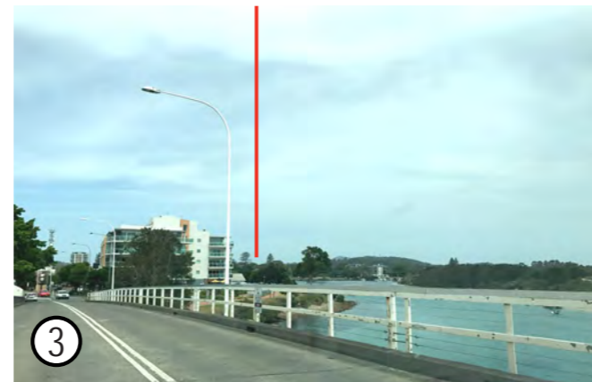
View east along Forster Tuncurry Bridge
