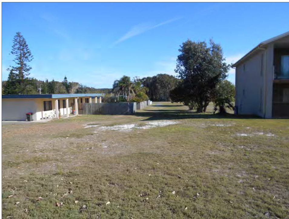
Figure 6.5 Existing holiday units and house facing west
