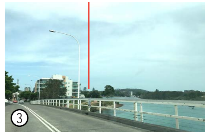
View east along Forster Tuncurry Bridge
