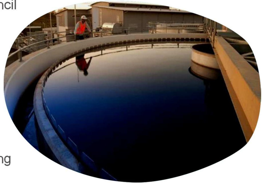
Bootawa Water Treatment Plant
